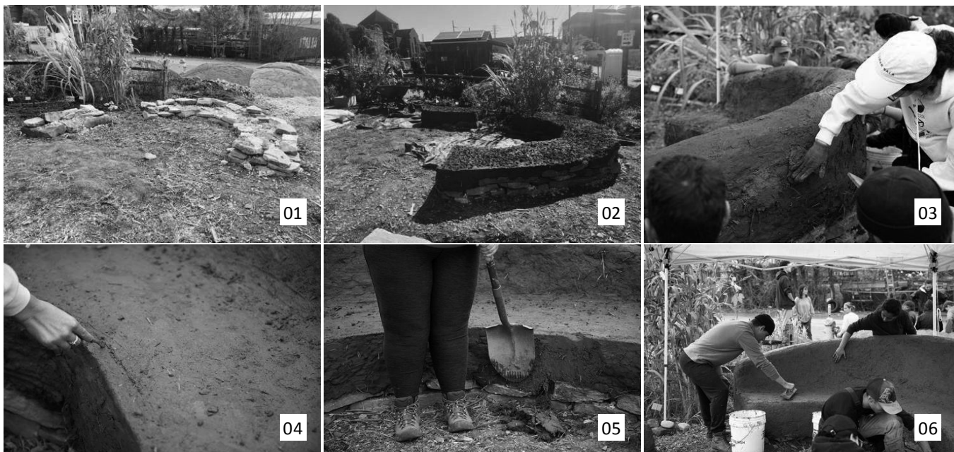
Figure 7: The steps for building and sculpting the cob bench and ottoman.
